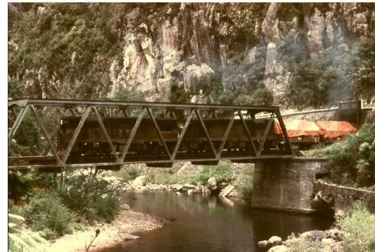
Figure 2: Railway bridge showing triangles and I beam
