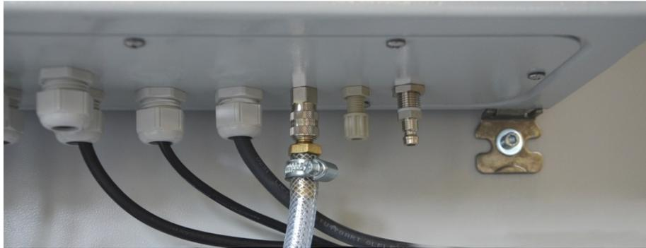
Figure 17: Connection for inert gas at the bottom of the safety module
