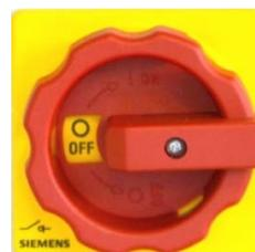
Figure 10: Gas detection system main switch (OFF position)
