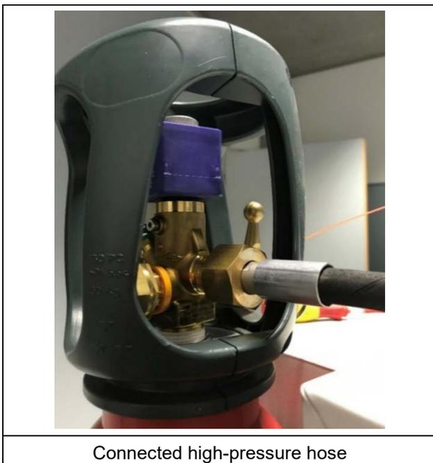
The union nut must be firmly tightened, otherwise leakage of CO<sub>2</sub> is possible.
