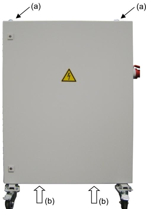
(a) Eyelets for lifting with a lifting crane or fork lifter
